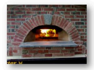
A test firing is the first time you bring your new oven up to baking temperature. If your goal is pizza, then this will be about 750F. Expect to drive most if not all of the leftover water from the masonry.
