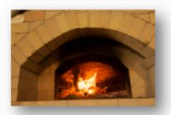
No matter what kind of oven you have, the mortar and other refractory materials need to be 'cured'.
